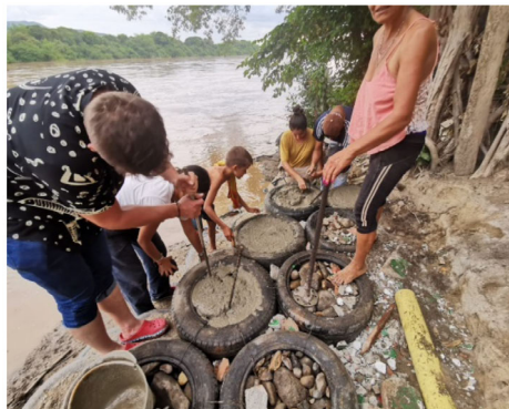
Figure 9. Wall construction process Source: Eduardo PeñalozaKairuz (2019)
