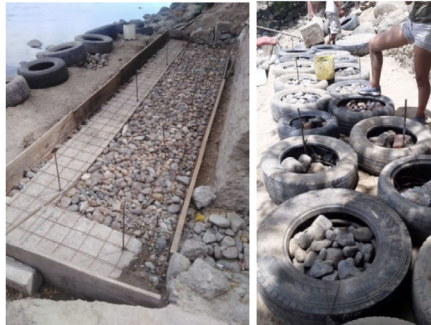
Figure 8. Wall construction start-up process. Source: Eduardo PeñalozaKairuz (2019)
