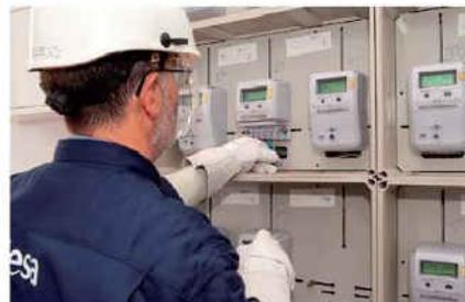
Figure 2. Placement of smart meters by an Endesa operator in the Smartcity in the framework of Málaga Project. Source: [3]
